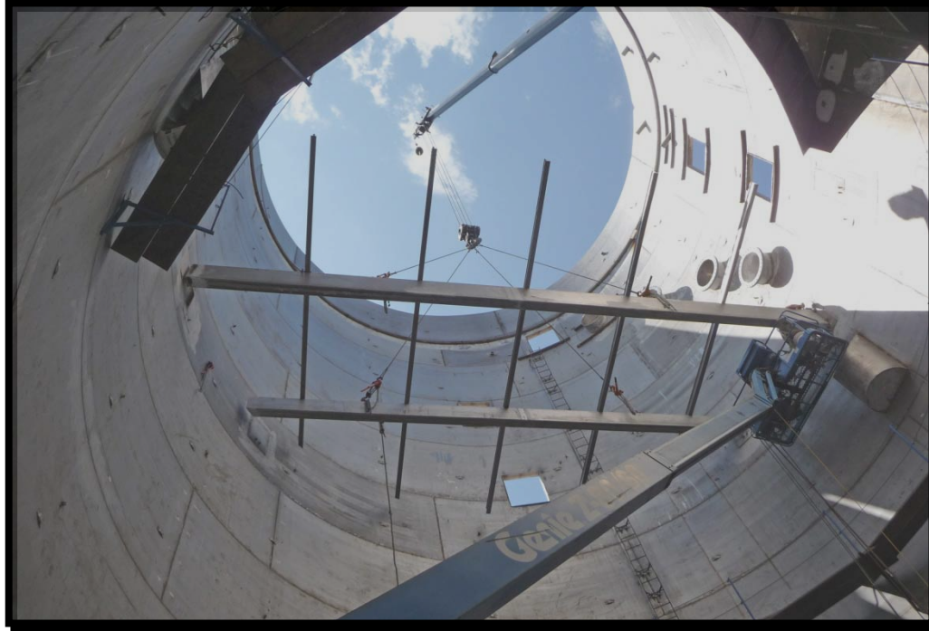
Maintenance Platform Installation Milton R. Young | Center, North Dakota
